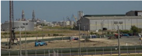
Construction site September 12, 2023.
