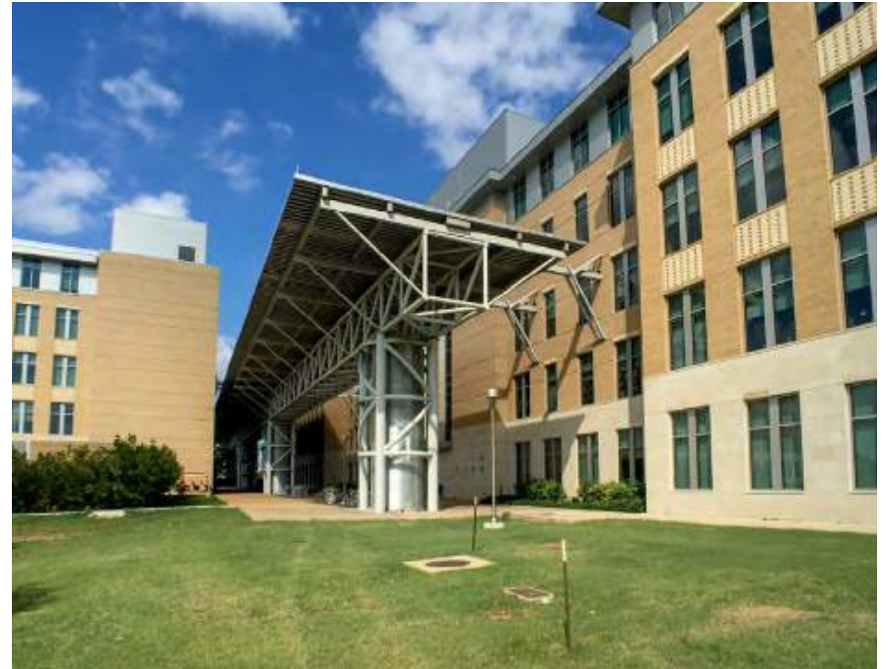
Rainwater collection at the TAMU Agriculture and Life Sciences Complex, photo by Patrick Creighton
