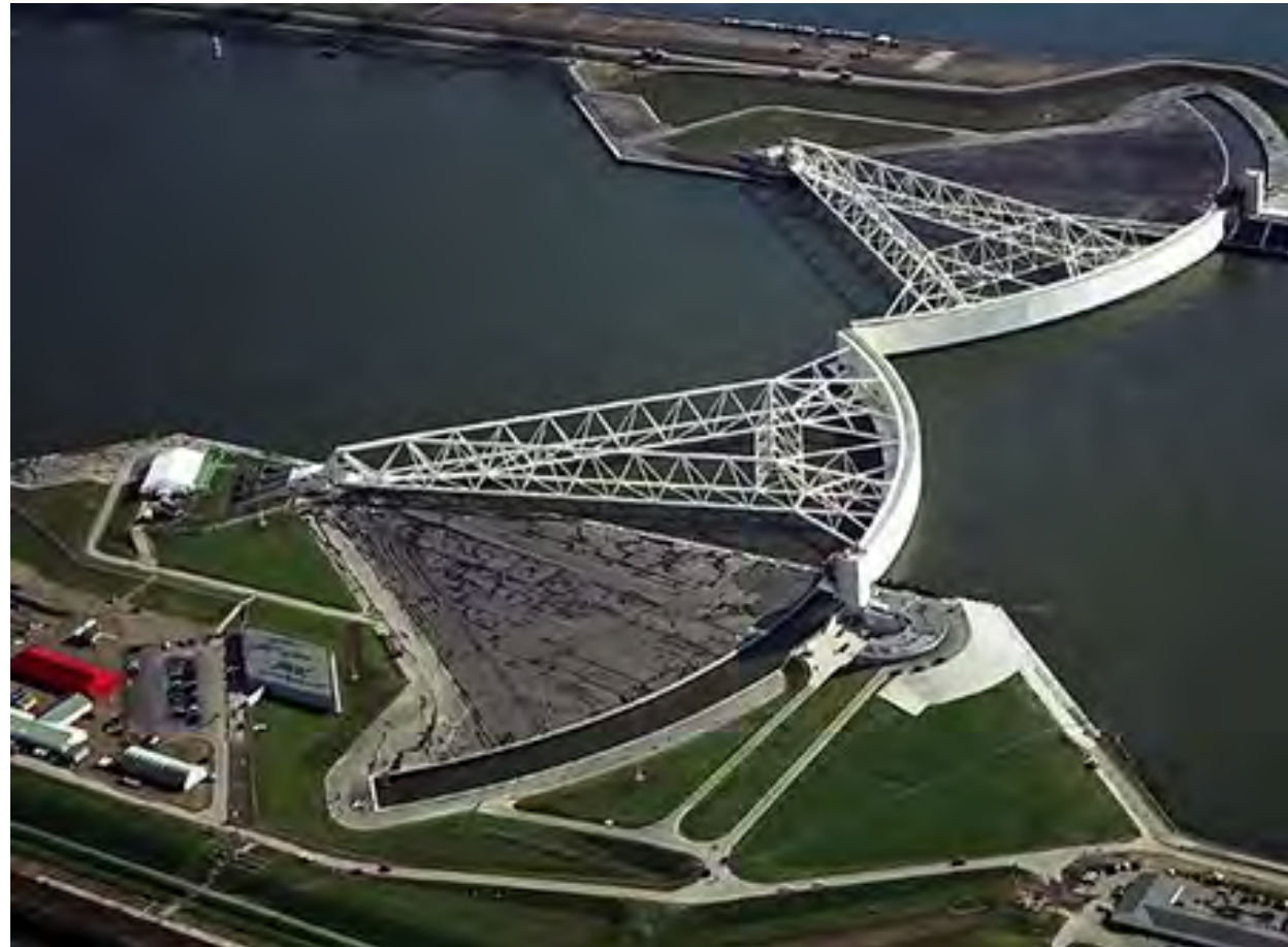
Flood gates at the Port of Rotterdam, similar to those proposed for the IJkdijk
